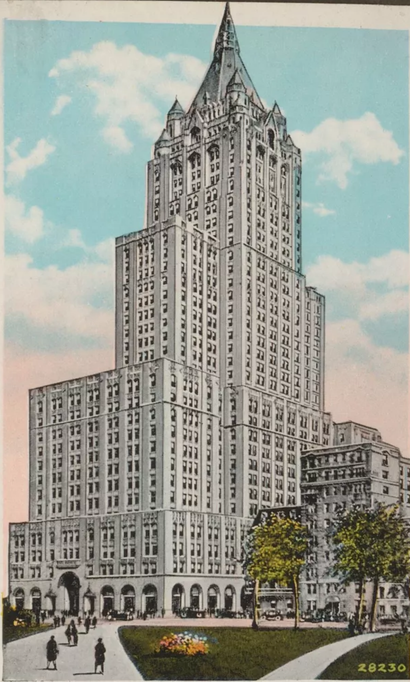
NEW YORK LIFE INSURANCE CO., NEW HOME, OFFICE BUILDING, NEW YORK.
